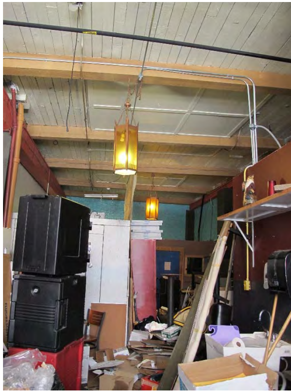
Fig. 70 – Interior, showing interior of third bay of north elevation; note painted-over skylights. This bay was originally part of the rear half of the building, but the restaurant expanded one bay westward.
