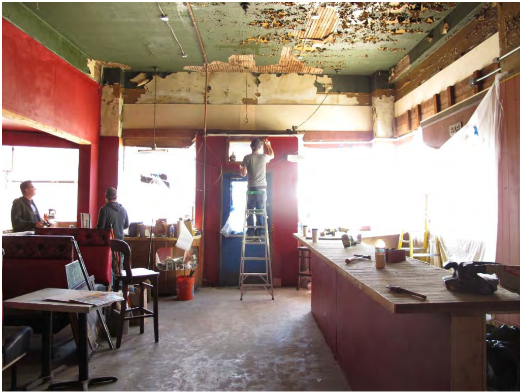
Fig. 66 – Interior, front half of building
