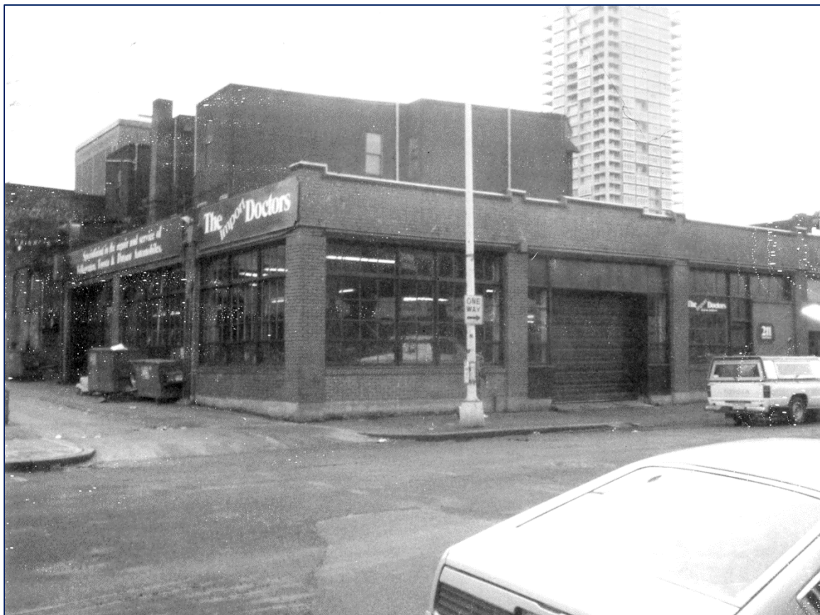
Fig. 21 – 1986 tax assessor photo, east and north elevations
