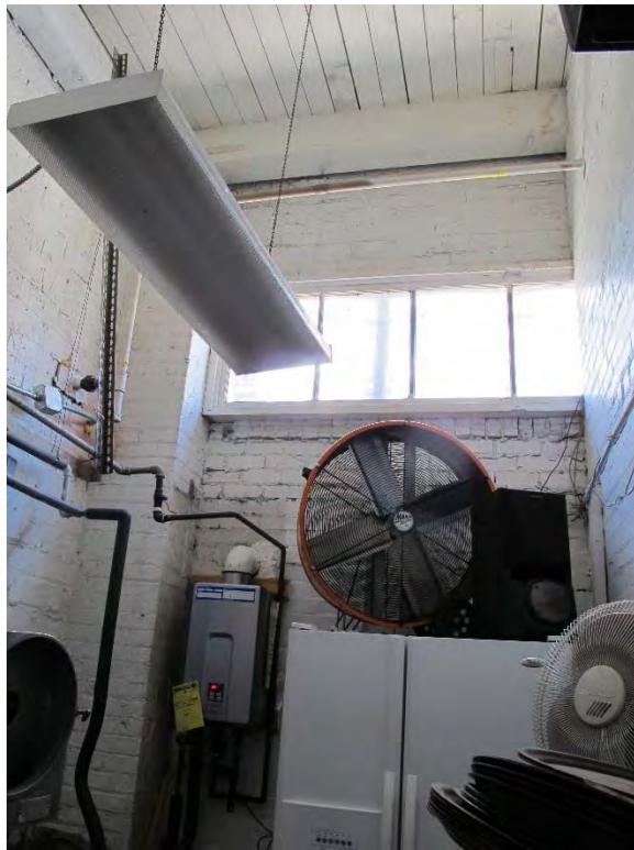
Fig. 71 – Interior, showing part of kitchen area against north wall fifth bay.
