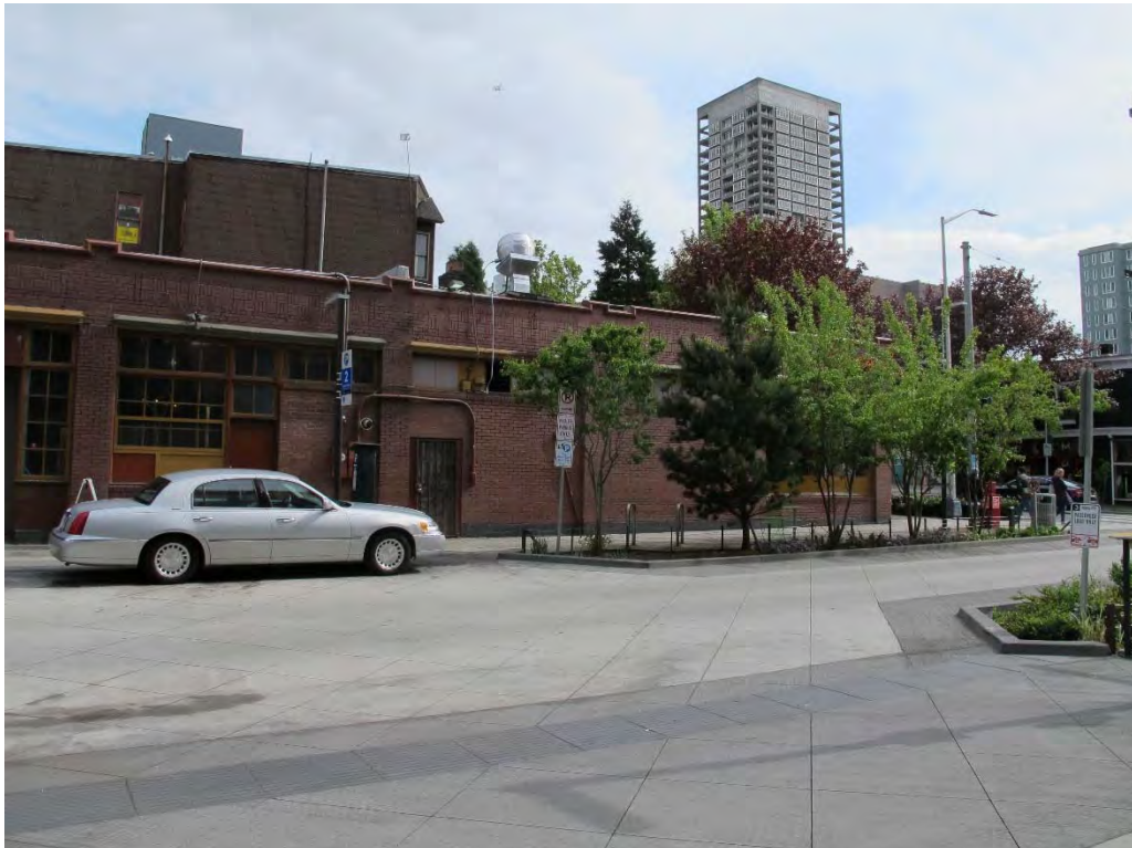
Fig. 57 – North elevation, third through sixth bays
