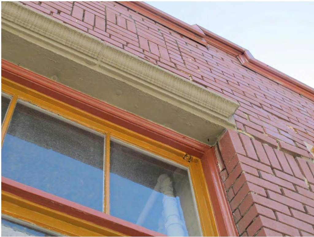
Fig. 64 – North elevation, detail of brick, cast stone coping and header, and window.
