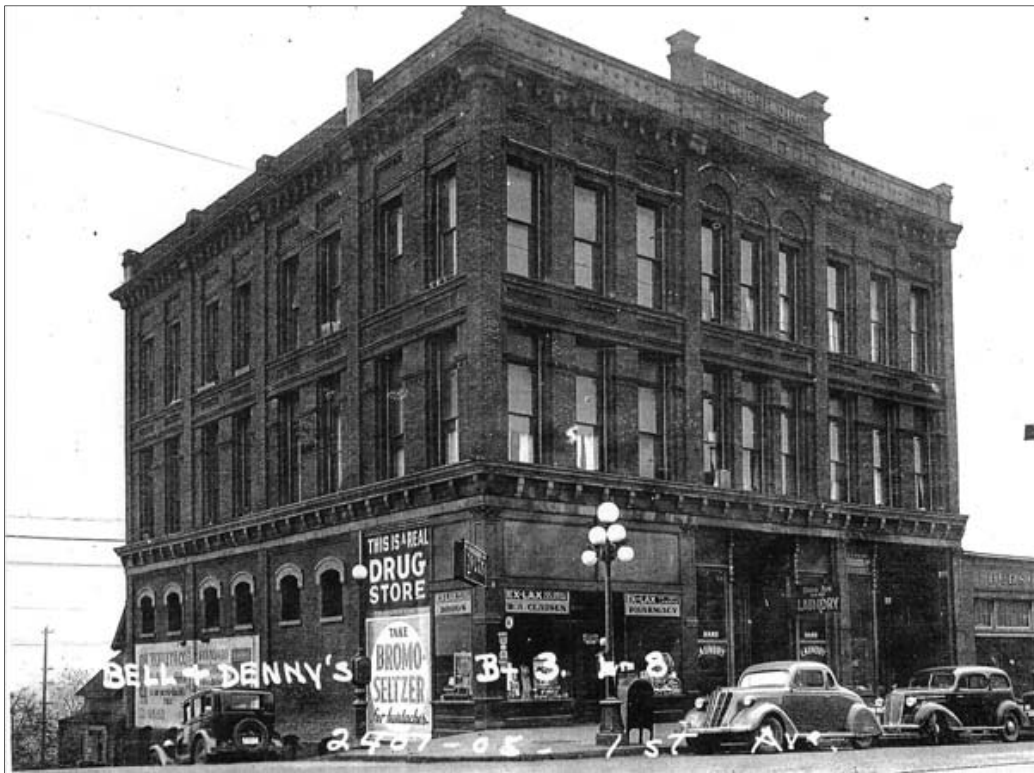
Fig. 6 – Hull Building, built 1889, at the northwest corner of First and Battery. (1937 tax assessor photo)
