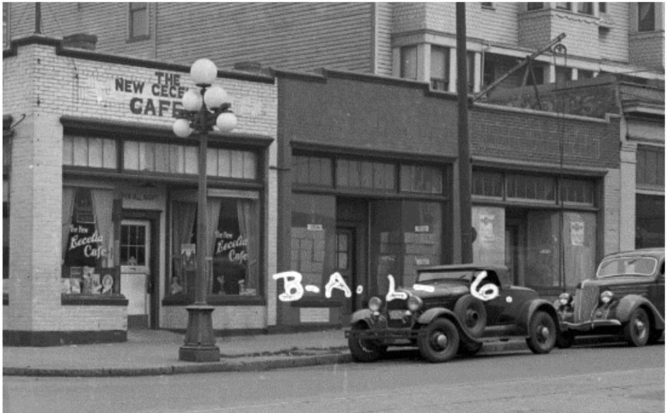
Fig. 16 – 1937 tax assessor photo, detail of west elevation
