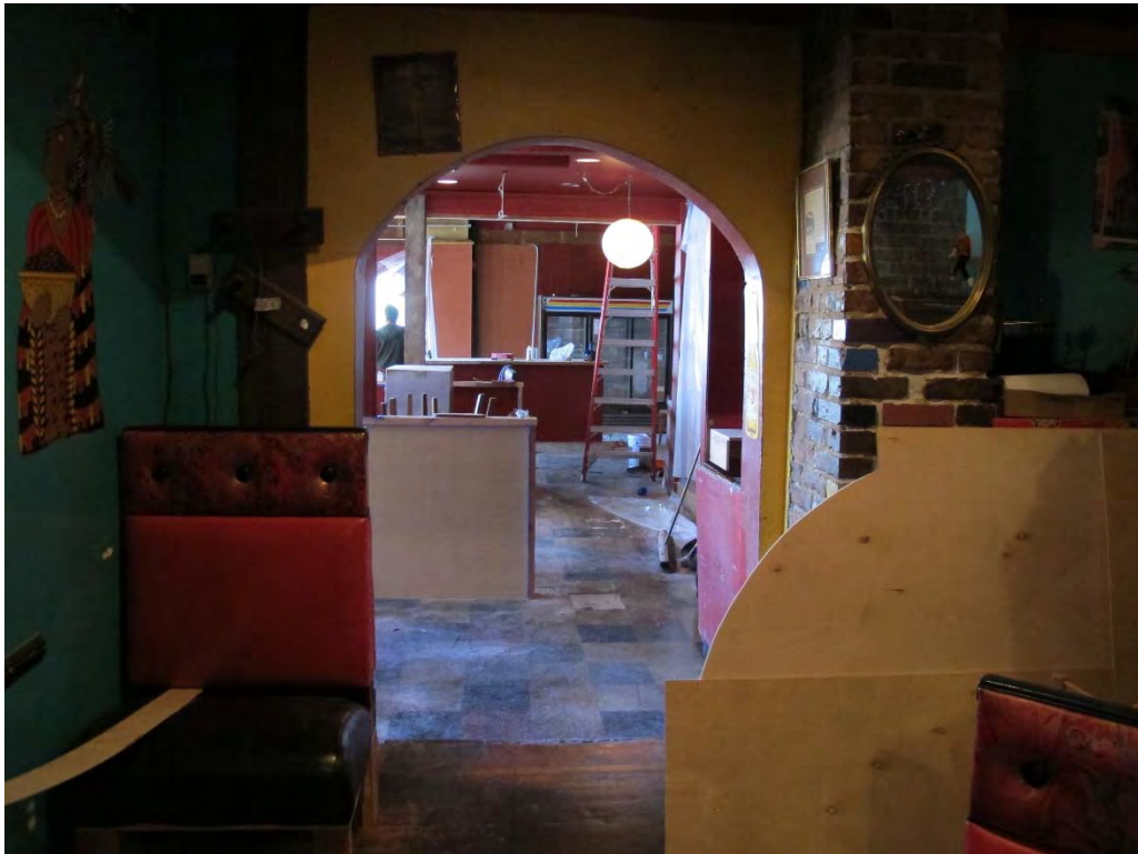
Fig. 69 – Interior, front half of building
