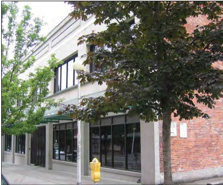
Fig. 32 – Similar Belltown buildings: 2106 Second Avenue (1919) (DON 2007 photo)
