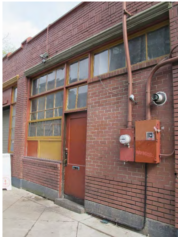
Fig. 59 – North elevation, third bay
