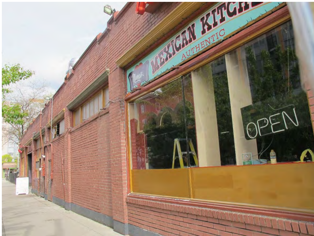
Fig. 62 – North elevation; closest bays shown are fifth and sixth bays
