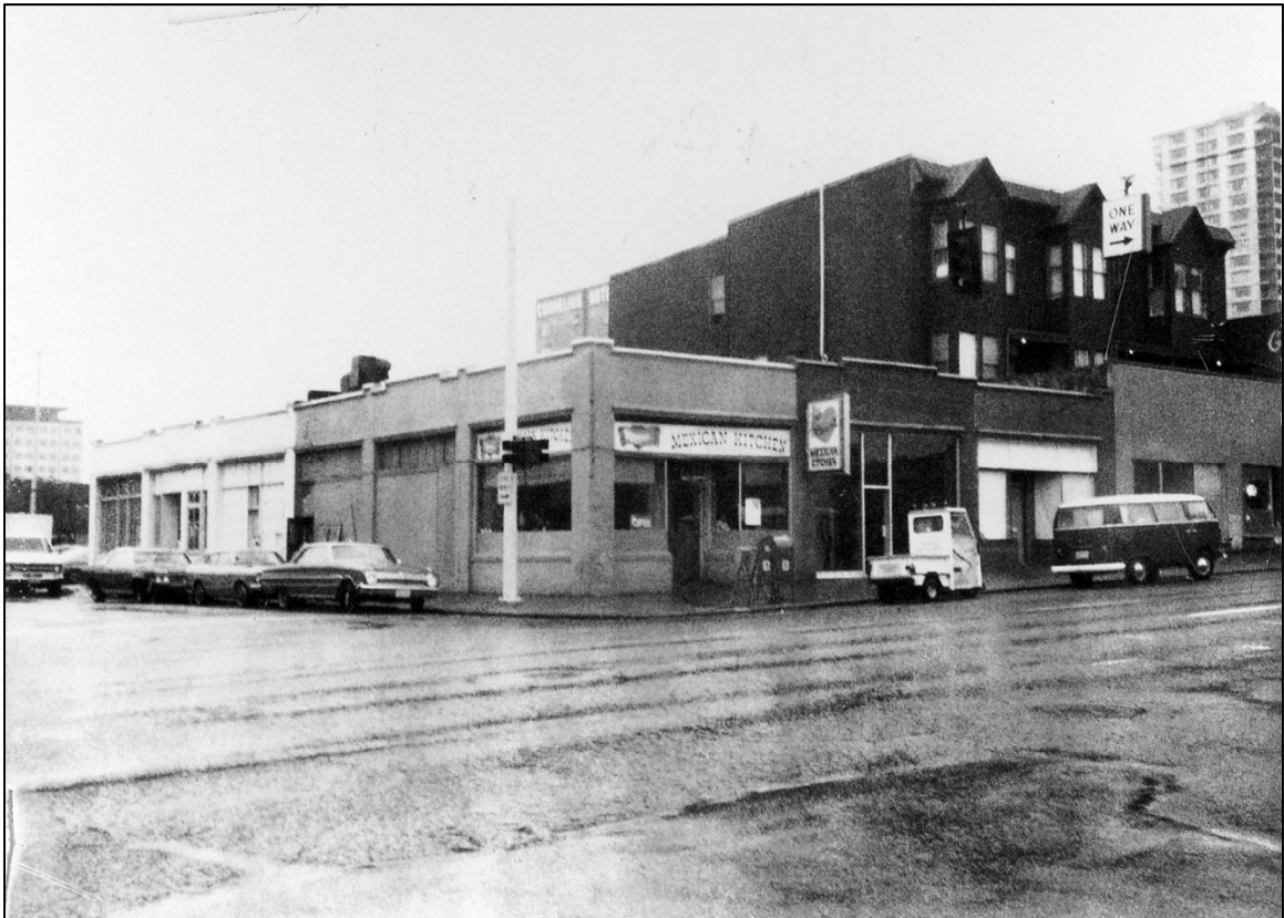
Fig. 23 – 1986 tax assessor photo, north and west elevations
