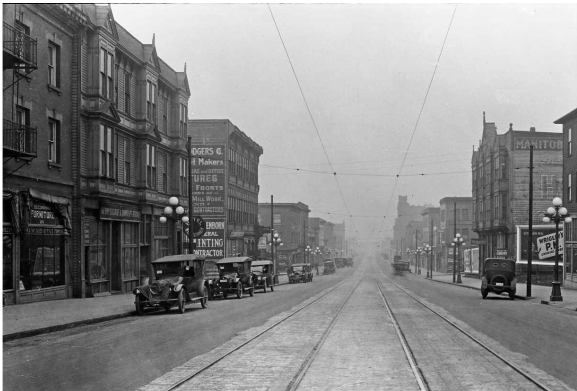
Fig. 12 – Circa 1915 view north on regraded First Avenue towards Blanchard; Bell Street in distance. (www.pauldorpat.com)
