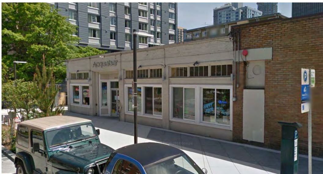
Fig. 28 – Similar Belltown buildings: 2230 Third Avenue (1924) Showing entire building (top), Third Avenue side (middle), and Bell Street side (bottom). Although the rear part of the building has been painted white to differentiate the commercial space, the entire building is actually one structure, (Google Streetview 2016)
