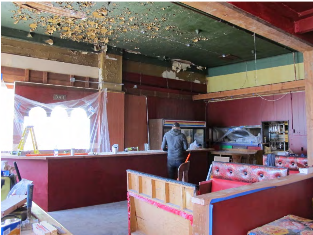
Fig. 65 – Interior, front half of building
