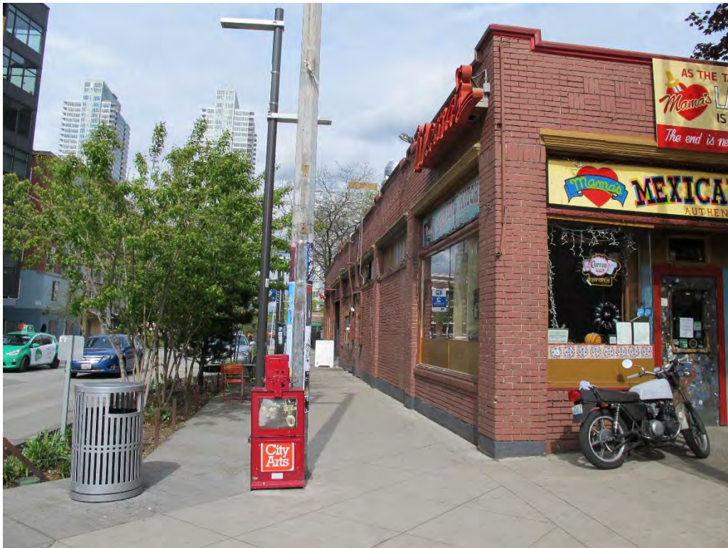
Fig. 61 – North elevation along sidewalk
